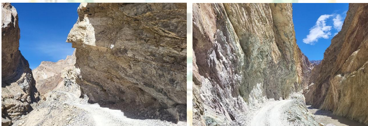
Fig.1: Nimu-Padam-Darcha Road, Ladakh Border Road Organisation (BRO). Critical sites of road widening using controlled blasting
