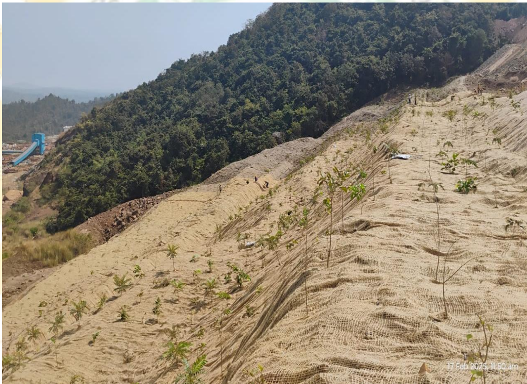
Fig. 5: Installed Geo Jute and plantation in a Slope area
