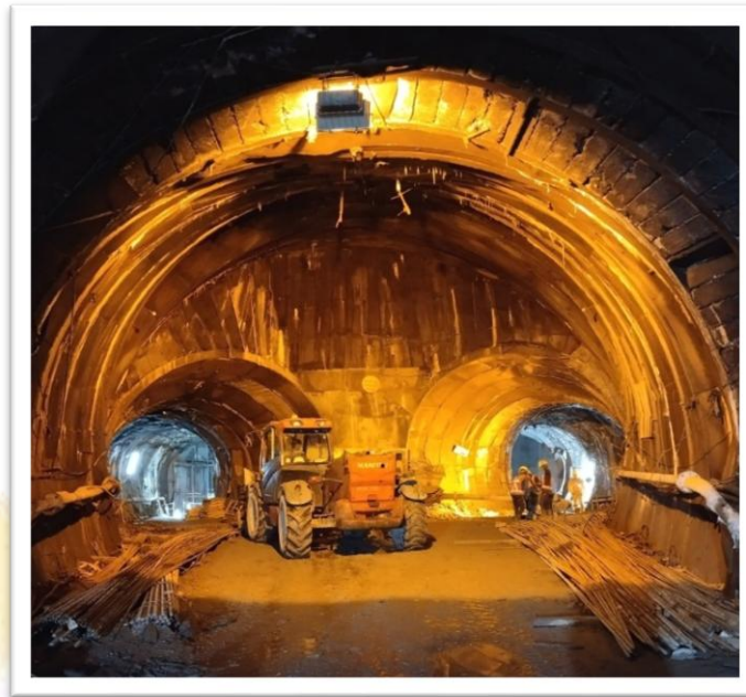
View of entry adits to powerhouse complex of VPHEP, Pipalkoti
