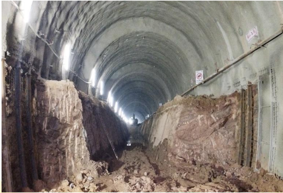
Fig.2: Ongoing benching work after completion of heading in tunnel T16
