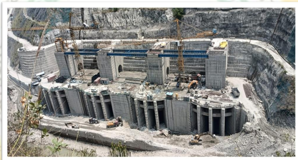
Site photograph of TRT Outfall Structures of Pump Storage Power Plant Project, Tehri showing completion of critical rock excavation and associated rock mass support
