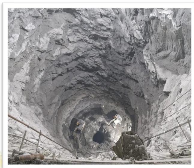
Shaft excavation using controlled blasting techniques at JSW-Kutehr Hydro Project
