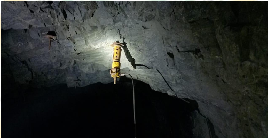
Fig.7: Anchorage testing of installed bolts conducted at the 16-17 VR development face at 174mRL.
