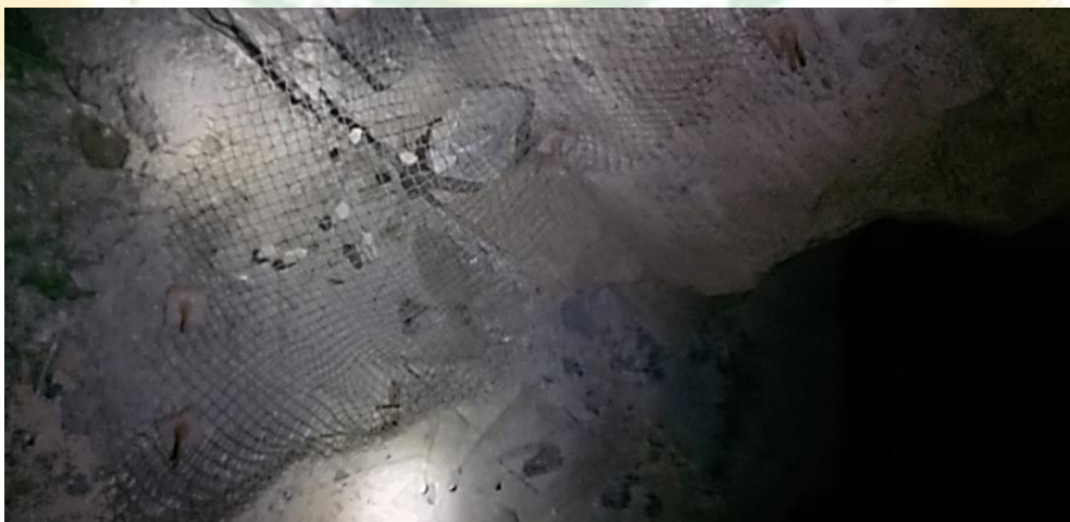
Fig.8: Roof condition near 14-16 VR at 120mRL.
