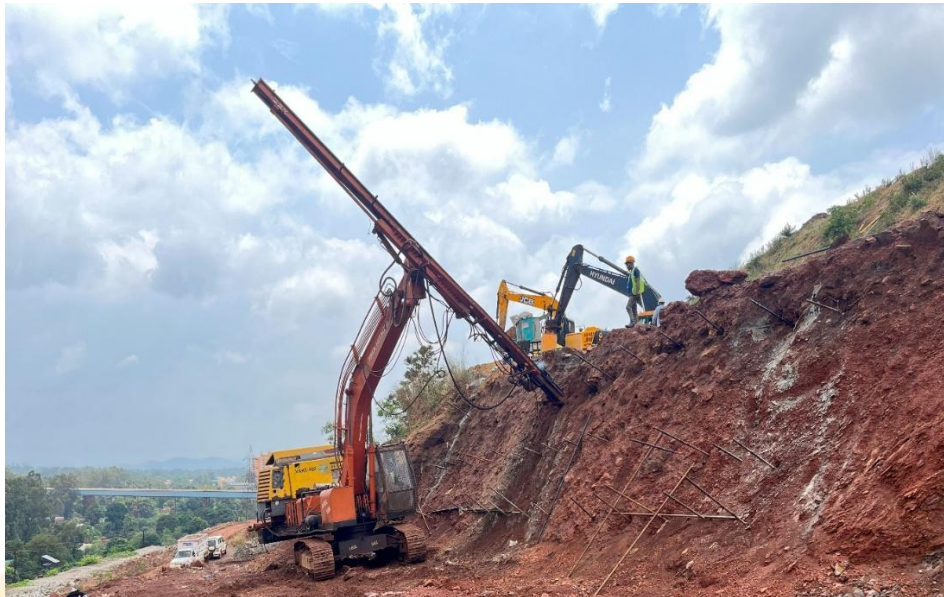
Fig. 4: Rock nailing work at slope site
