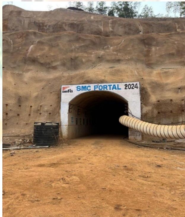
Fig. 3: Ground improvement by soil nailing surrounding to portal for slope stability
