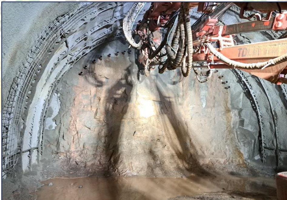
Fig.1: Face advancing with pipe roofs at BBB in tunnel T14
