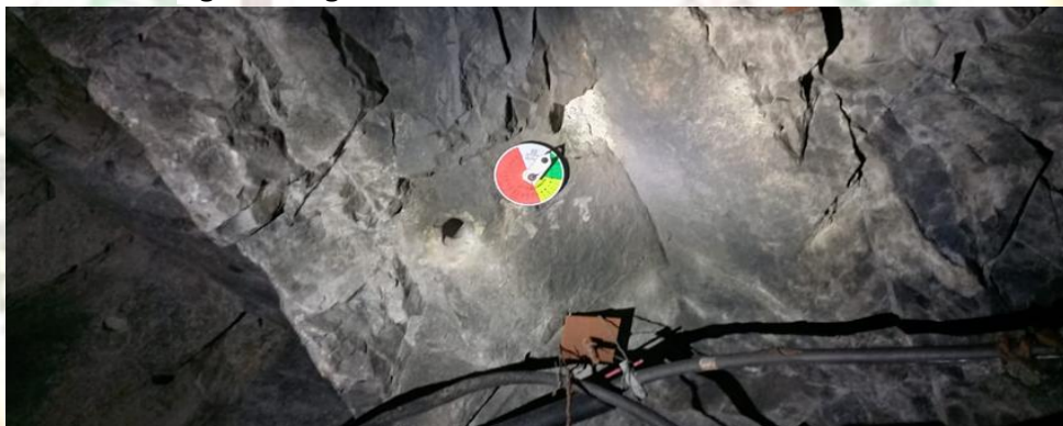
Fig. 6: Rotary telltale installed at the S-V-B-14-16 stopes drill junction at 174mRL.
