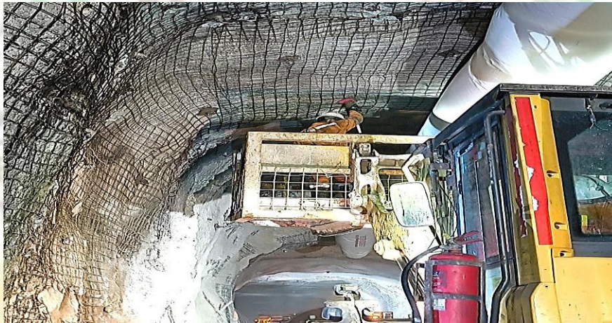
Fig. 13: Anchorage testing of Rock Bolts at location -380L NN352.
